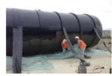
Kebu Bitumen-Tape GW/HT is suitable for post-wrapping of factory-wrapped pipes or pipe fittings as well as for wrapping of large-diameter pipes and vessels and complies with the scope of application specified in DIN EN 10300, Annex J7. The coating of large-diameter pipes and containers must be double-layered in accordance with DIN EN 10300, Annex P6. Together with the liquid adhesive Kebusol-Primer HT it forms an effective corrosion protection system.
